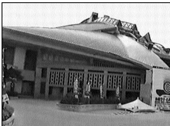
Okinawa Prefecture Budokan
